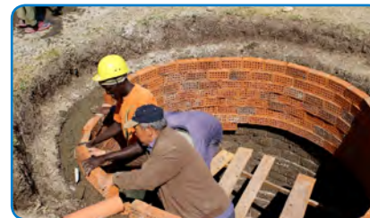
On-job Training on the Construction of Rainwater Harvesting Storage, Kenya, 2014
