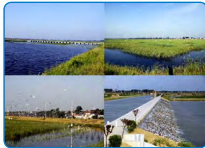
Yanlon Lake Water-Source Project in Yancheng City, Jiangsu Province
